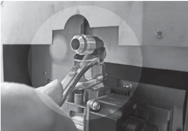
2. Install alternate elbow (not supplied).
