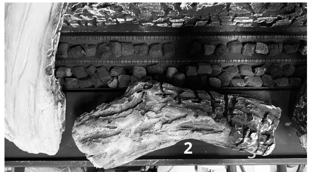
Top view—Log 2 installed
