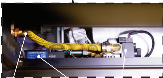
Gas Line Receiver Control Valve
