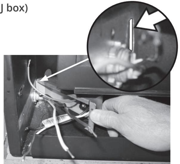
4. Connect the corresponding wires and cap them with wire nuts.
