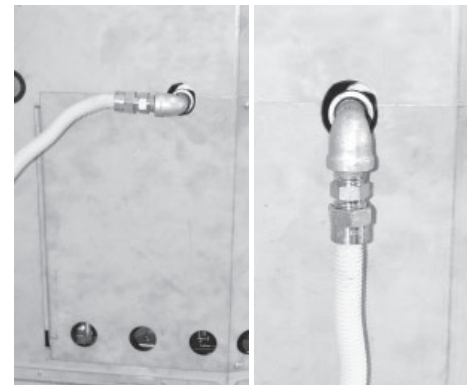
Flex connector redirected using two elbows.
