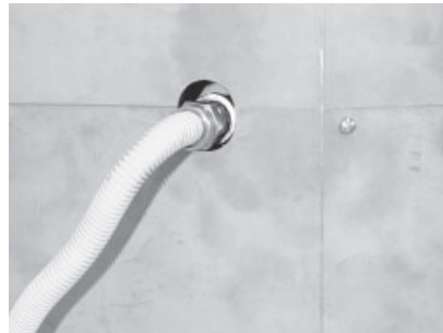
Flex connector redirected using one elbow.
