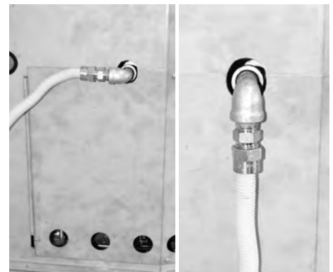
Flex connector redirected using two elbows.
