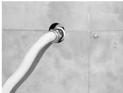
Flex connector redirected using one elbow.
