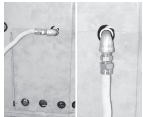
Flex connector redirected using two elbows.
