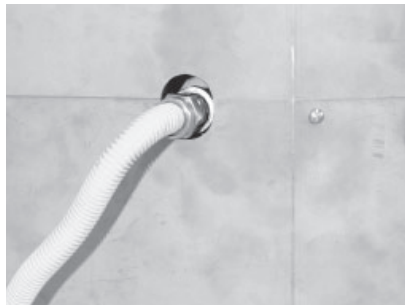
Flex connector redirected using one elbow.
